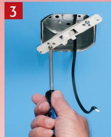
3 Mount the bracket to the existing box using screws provided.
