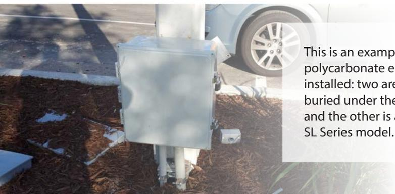
This is an example of three polycarbonate enclosures installed: two are L Series units buried under the landscaping, and the other is a pole-mounted SL Series model.
