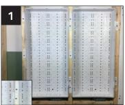
Place enclosures between studs side-by-side.
