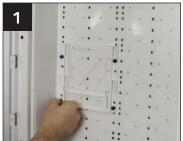
Insert push pins to affix SMS to the Media Distribution Enclosure.
