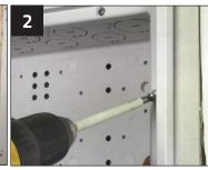
Install frame and lid using the provided No.8 screws.
